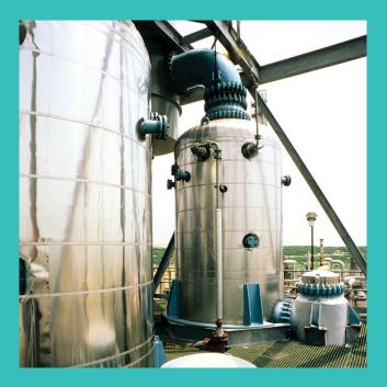
PURIFICATION — Processes for Sulphuric or Nitric Acid contaminated with volatile or oxidizable contaminants are purified in our purification columns prior to vacuum concentration. Minimization of energy use and maximizing removal efficiencies take centre stage. Inorganic contaminants are removed by (membrane) filtration or precipitation.
