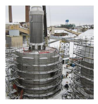
Worley Chemetics also specializes in the design, supply and installation of replacement gas/gas heat exchangers on existing plants.
