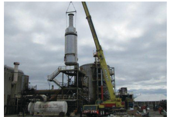
Preheat Exchanger being installed
