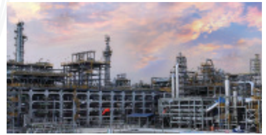
CORE-FGD™ installation, South East Asia
